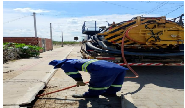
RUA I - SEWERJET
