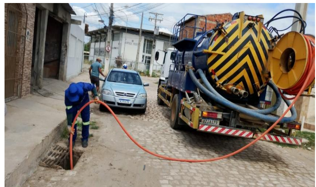
RUA M - SEWERJET
