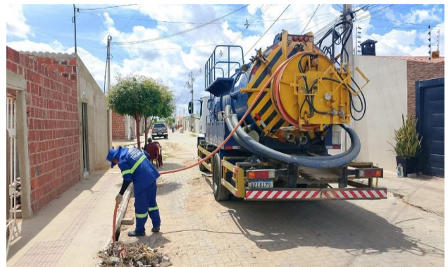
RUA A - SEWERJET
