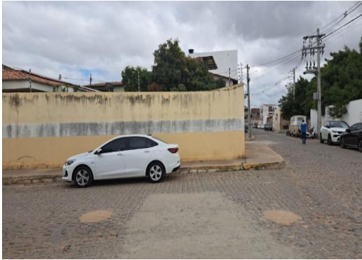
HOSPITAL REGIONAL - TAPA BURACO PARALELO
